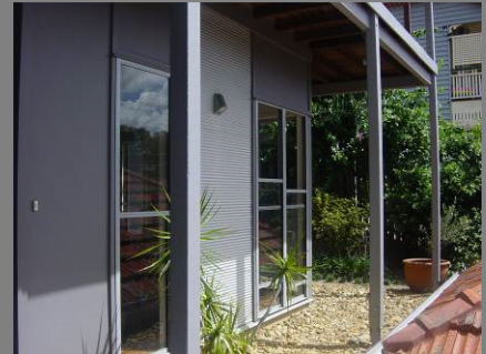
Reno, Toowong. Lift and build-in. Note that contemporary materials were used at the lower level to break up the elevation of the house.
