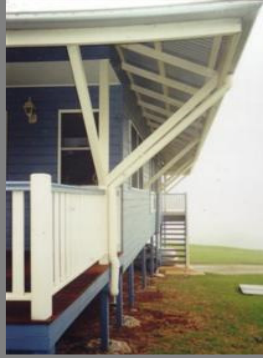
Large propped overhangs protect against sun and rain
