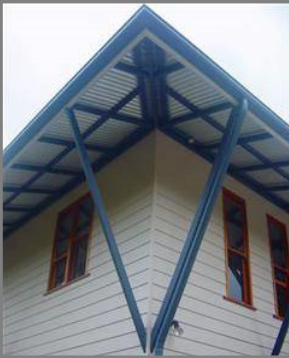
Large propped overhangs protect against sun and rain
