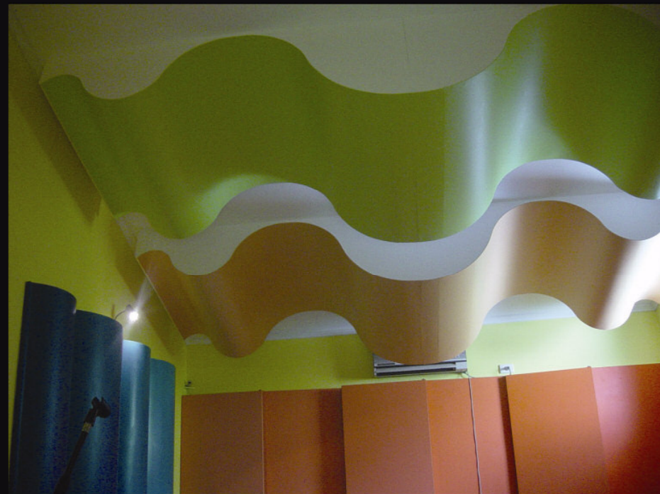
baffling used as sound control throughout the studio
