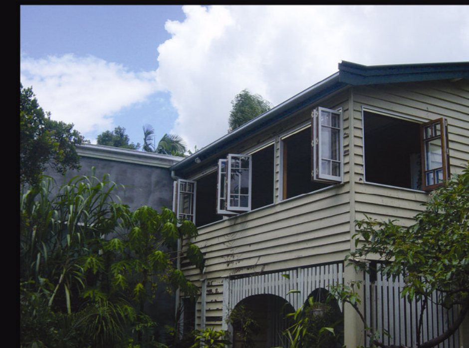
northern side of studio against the existing house
