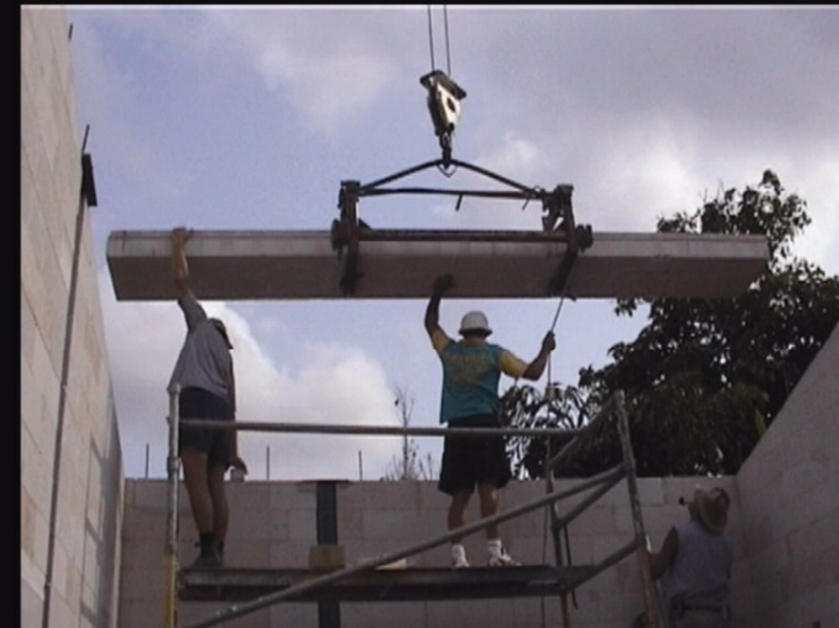
inserting the hebel panels during construction
